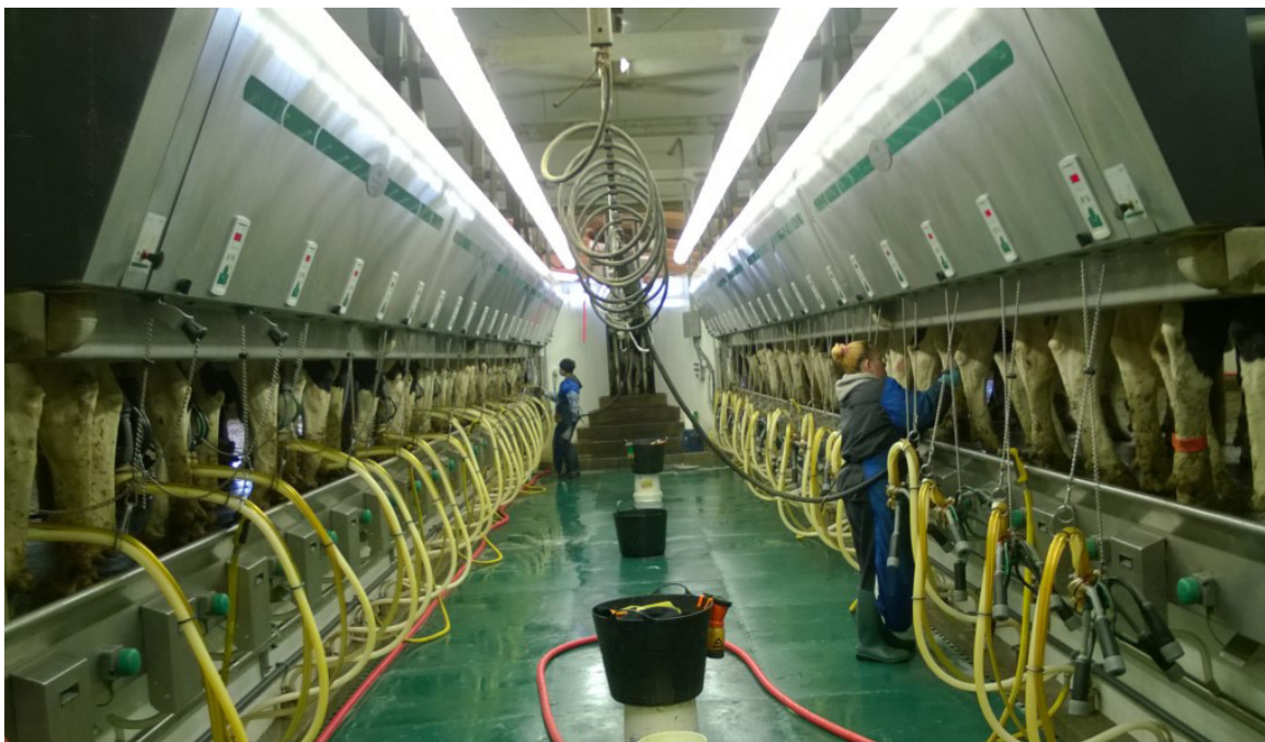
Parallel parlors feature an elevated platform as well, but are angled at 90-degrees facing away from the operator. Milkers access the udder from the rear legs which can make sanitation and unit attachment difficult.
